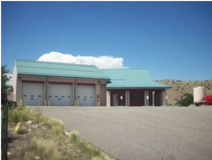
Placitas Fire Station
